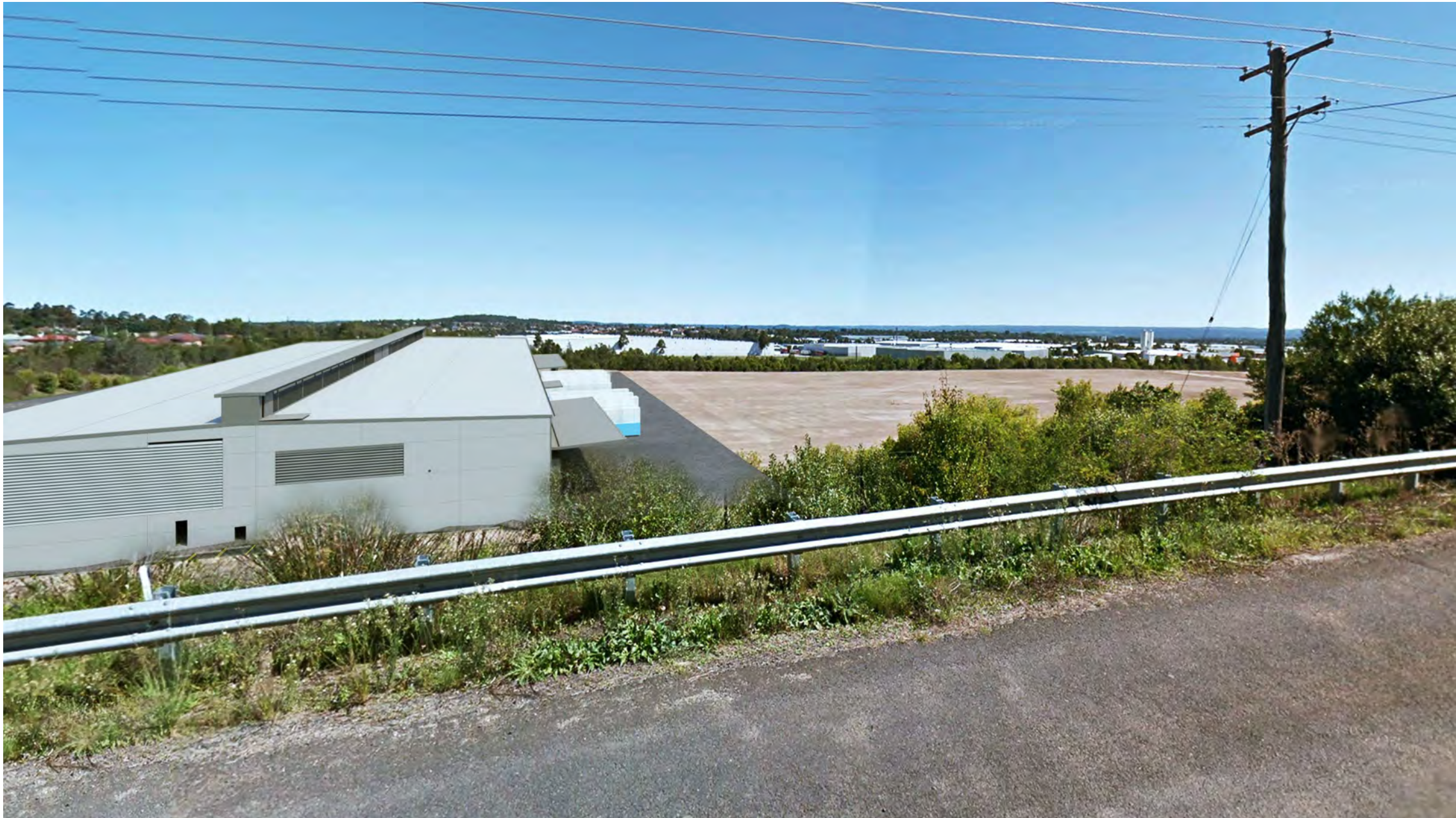
LEFT : VIEW RECEPTOR 4 EXISTING VIEW FROM TURNER ROAD
